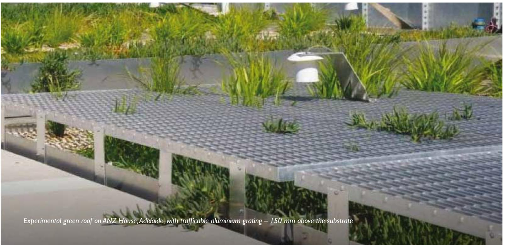
Experimental green roof on ANZ House, Adelaide, with trafficable aluminium grating – 150 mm above the substrate
