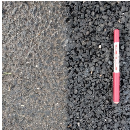
Figure 4 Permeable asphalt, Harris St, North Melbourne
