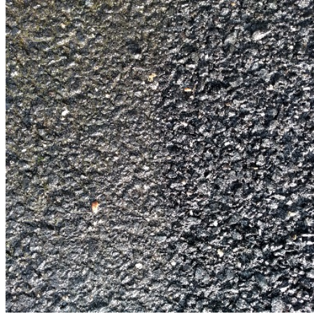
Figure 2 Permeable asphalt, Eades Pl, West Melbourne
